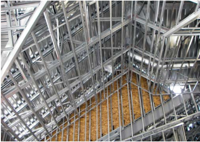
Using cold-formed steel as part of a building's structural system can reduce total construction costs.
