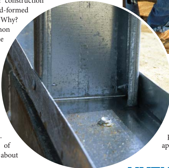
Cold-formed steel is an effective option for load-bearing walls.
