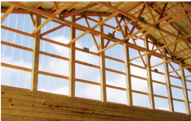
Clear polycarbonate allows the greatest amount of light transmission. However, since the light is not diffused, as it would be in a translucent panel, it can create a "hot spot." PHOTO COURTESY OF PALRAM.
