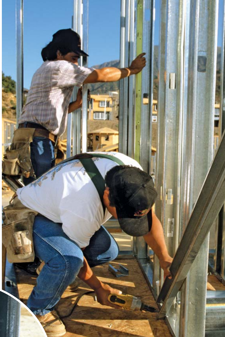
Cold-formed steel is an effective option for load-bearing walls.
