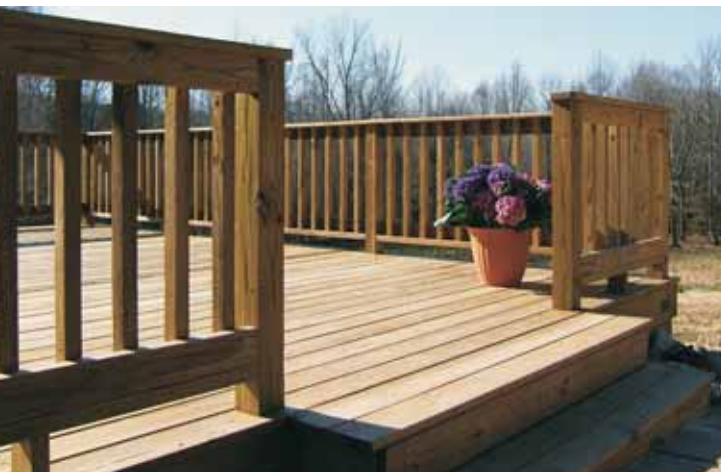
Exterior Fire-X® used in the wildland-urban interface (WUI) for decking to comply with ignition-resistant material requirements. Photo courtesy of Hoover Treated Wood Products.
