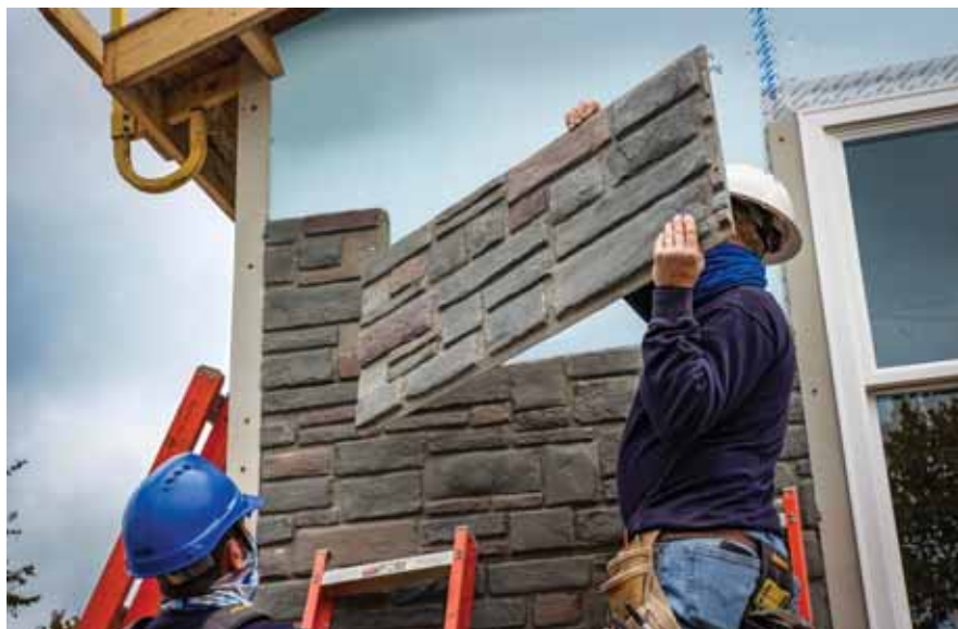
Qora® Cladding provides the look and feel of real stone with less labor-intensive installation. The resin-based cladding is Class-A rated for two-hour wall assemblies. Photo courtesy of Arcitell®.
