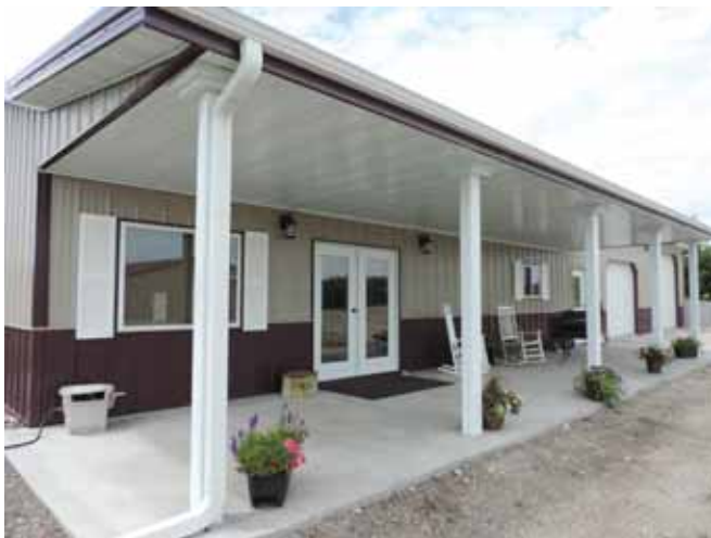
Porches are a common enhancement to residential post frame. Photo courtesy of K-Construction.
