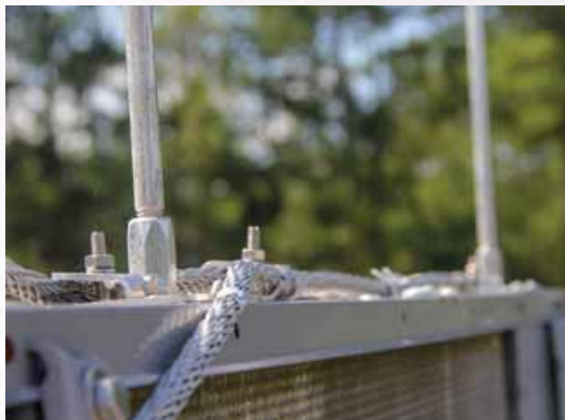
Any system on the roof can have lightning protection added to it. Fittings and attachments can be placed on cupolas, weather vanes, and fan units to give them the needed protection from lightning strikes. Photo courtesy of LagPro.
