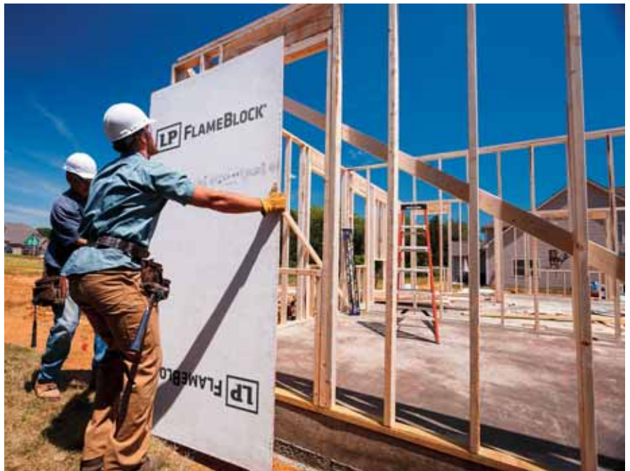
LP FlameBlock®, OSB coated in a non-combustible substance, can limit damage from exterior fire threat to the siding and sheathing. Photo courtesy of Louisiana Pacific.
