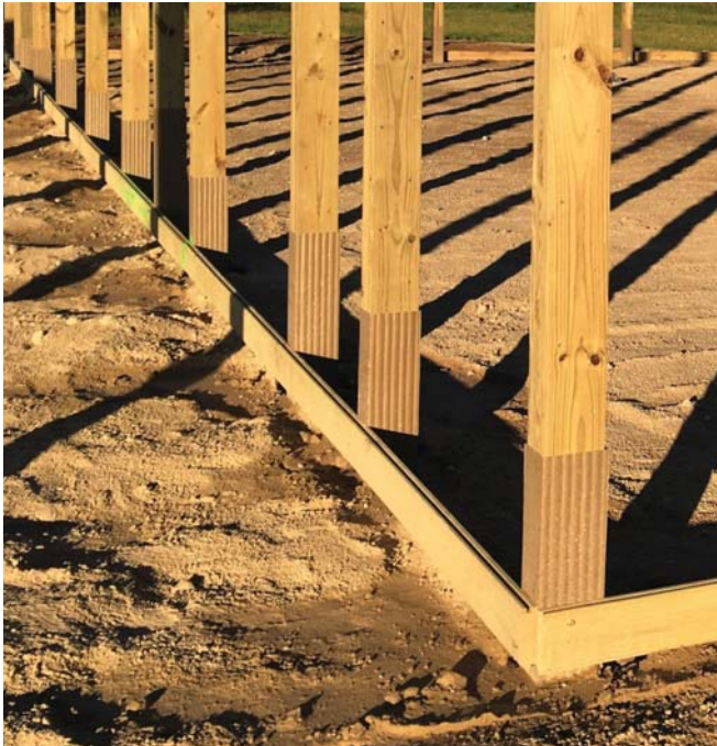
Post Protector is a physical barrier made from a specialty high-density polyethylene that is commonly used in landfill liners. Photo courtesy of Post Protector.
