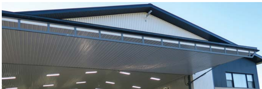
55 x 18 door on hangar condo. PHOTO COURTESY OF POWERLIFT DOORS.
