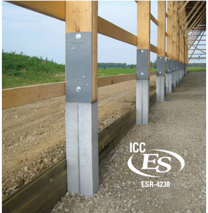
Perma-Column elevates the wood posts out of the ground with pre-cast concrete and steel brackets. Photo courtesy of Perma-Column.
