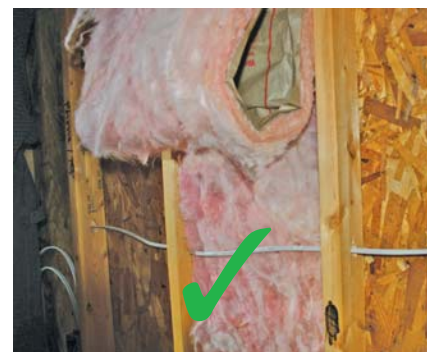
(Above) Installed to the required density and thickness to achieve the labeled R-Value.
