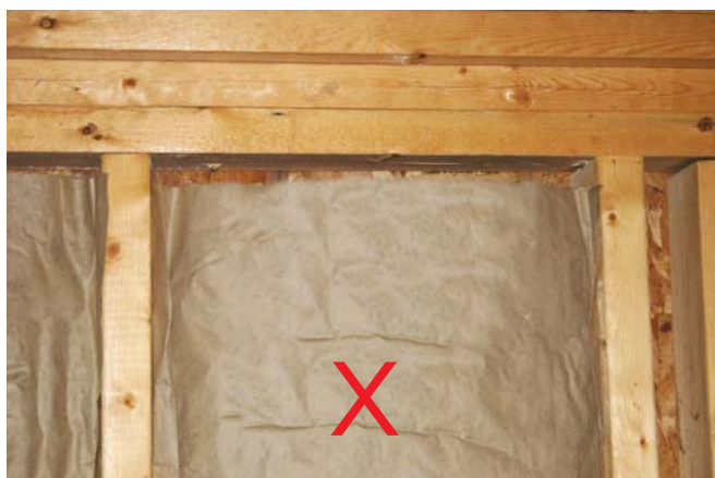
(Above) NO GAPS/VOIDS —Insulation is in full contact with all sides of the cavity, side to side and top to bottom. All photos courtesy of Owens Corning.
