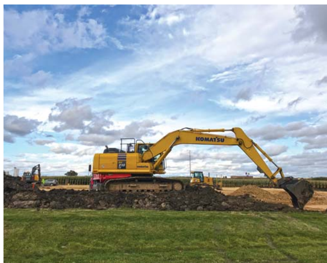
Properly preparing the build site is an important step to a successful project.
