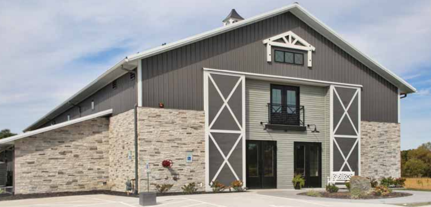
Courtesy of Greiner Buildings
