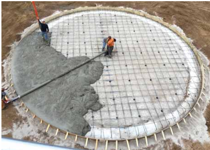
Roller screeds that can easily change spin direction allow operators to screed clockwise or counterclockwise during the pour, eliminating the risk of a cold joint. PHOTOS COURTESY OF CURB ROLLER MANUFACTURING
