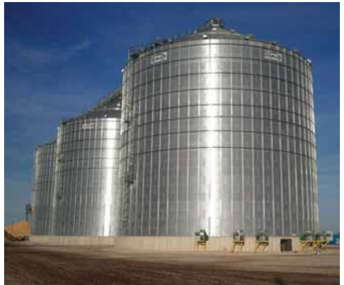
Bins from Sukup Manufacturing feature precision-engineered 4" wide corrugated high-strength 50,000 psi yield strength, 70,000 psi tensile strength galvanized steel sidewall sheets to provide greater vertical load carrying capacity. PHOTO COURTESY OF SUKUP MANUFACTURING CO.
