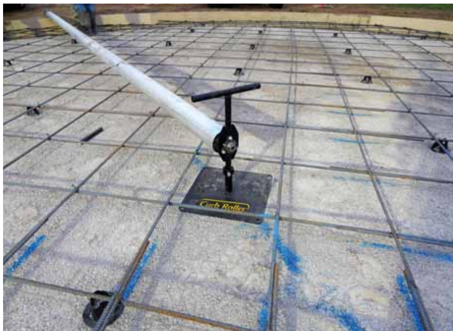
A pivot kit minimally consists of a metal stake fixed to a weighted base, which is affixed to the center of the work area. The kit can be used as a guide to frame out the circular pad and gives users the ability to attach one end of a concrete screed to the center stake and control the screed from the other end.
