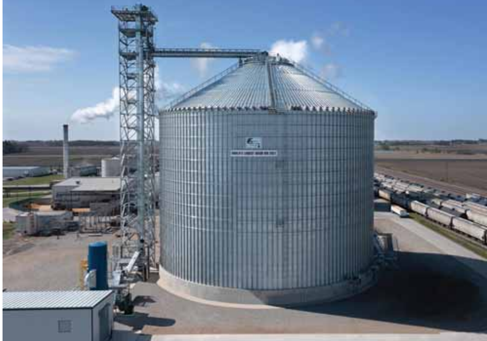
Sukup Manufacturing designed this 2.2 million bushel grain bin for Golden Grain Energy, LLC in Mason City, Iowa. Bin construction was completed in June, and is currently the world's largest free-span grain bin. PHOTO COURTESY OF GOLDEN GRAIN ENERGY.
