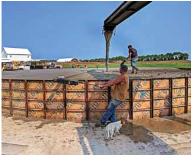
Battery powered roller screeds are typically lighter and more easily maneuvered than alternative methods. The ability to change spin direction at the push of a button allows operators to effortlessly screed clockwise or counterclockwise.
