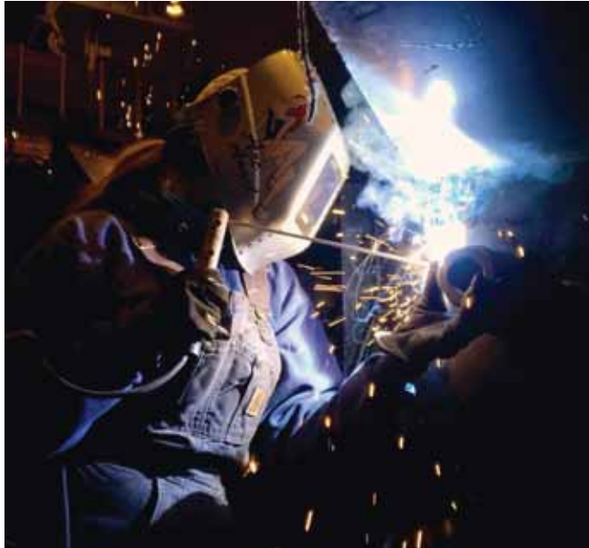
Hudson welding nuts onto a rotor for a turbine refurbishment at Bear Swamp hydroelectric plant in Massachusetts.
