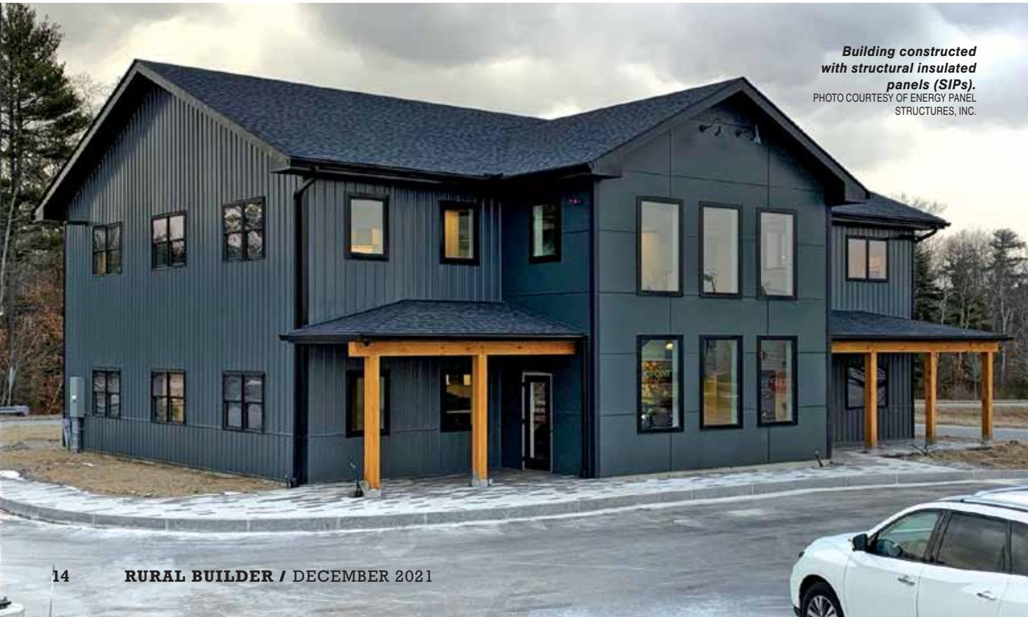
*Building constructed with structural insulated panels (SIPs).*
