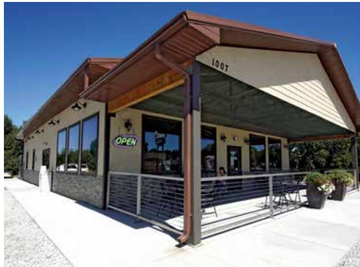
*SIPs were used to build this commercial space. As a result, the owner will see energy savings throughout the life cycle of the building.* PHOTO COURTESY OF ENERGY PANEL STRUCTURES, INC.
