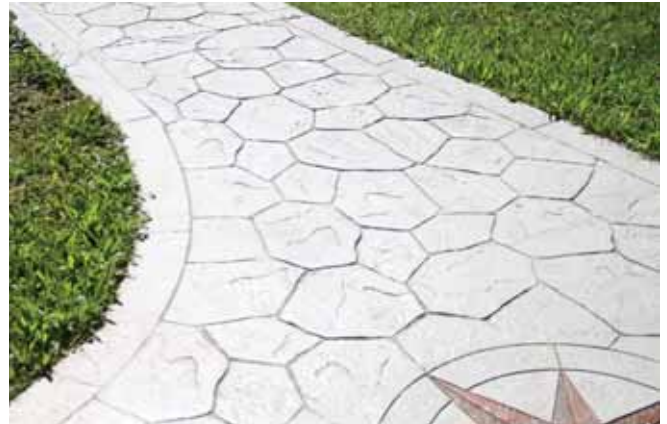
Color in the cement with release color on top; plus acrylic based stain on compass.
