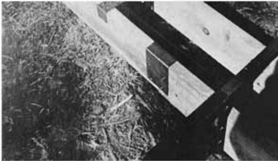
By making support tube 48 in. long, the support gussets handle 18-in. wide situations, as shown here, and still have some adjustments left.
