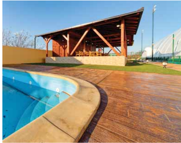
Wood Plank Texture with one color in the concrete and one over the top.
