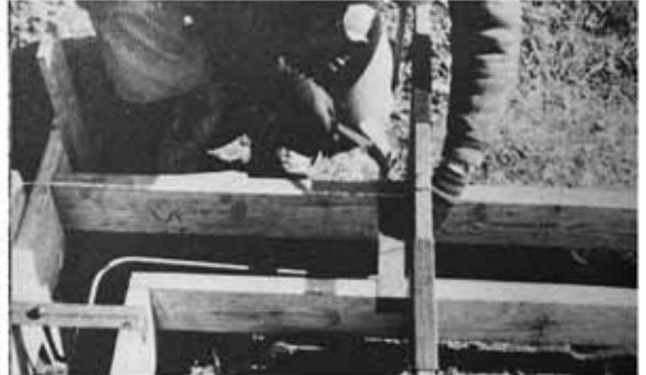
Young modified this form for use in his business. He uses two sizes of square steel tubing that slide together making adjustable support gussets.
