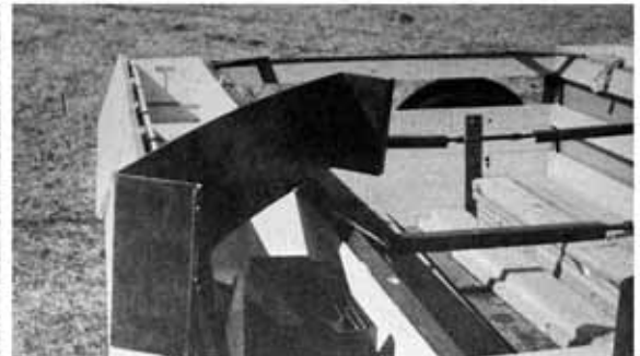
He cuts forming lumber to fit his trailer. To eliminate unloading and reloading at shop, he built boxes on side to carry the cross members.
