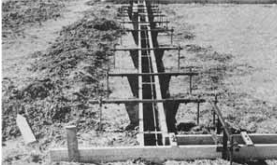
Estel Young saw the steel cross member, a technique developed by Schuh Brothers, Hoyt, Kan., used for forming the curtain wall foundation.
