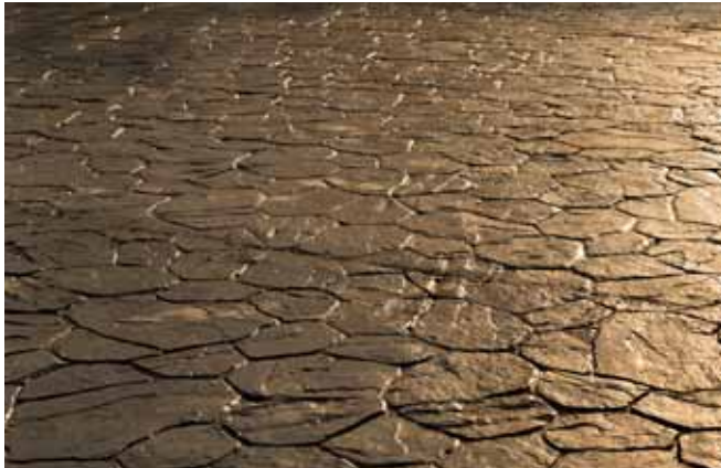
Color in the cement with release color on top.
