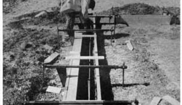
Adaptability's built into Young's system. When necessary, crew members make up some steel splice plates that firmly hold the ends together.
