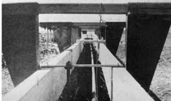
His crew cut and welded cross members to lay foundation. Steel templates hold anchor bolts, and a wire method supports reinforcing rod.
