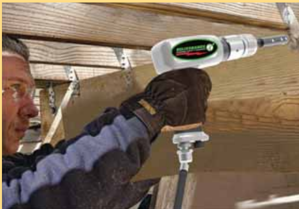
For driving bulk nails and spikes, a pneumatic “mini jackhammer”-type nail driver will accommodate many fastener types and sizes. PHOTO COURTESY OF DELIVERANCE POWERED SAFETY HAMMERS.
