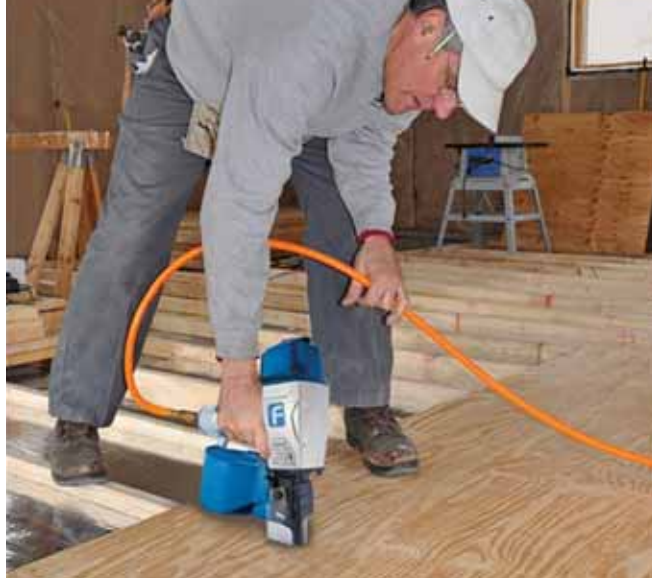
Installing subfloors with the pneumatic SCRAIL® SubLoc® PRO from BECK America. PHOTO COURTESY OF BECK AMERICA.
