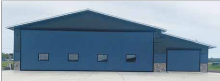
The main Schweiss Doors hydraulic hangar door is 54 feet by 16 feet, 9 inches and an adjacent storage room/garage door measures 13 feet, 3 inches by 8 feet, 11 inches. Four well placed windows on the large hangar door and front hangar windows bring a large amount of natural light into the hangar.
