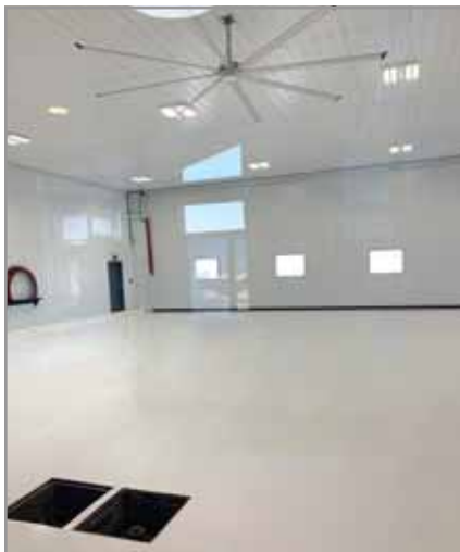
An energy efficient "Big Ass Fan" is the answer to effective airflow solutions within the hangar. Two floor drains help to keep the hangar floor immaculate.
