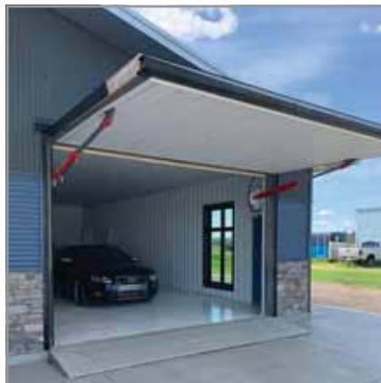
This part of the hangar building is used as a storage area and garage. The hydraulic door is 13 feet, 3 inches by 8 feet, 11 inches. Both doors have their own remote openers. Notice the beveled concrete at the entrance that keeps rain from entering the garage and hangar.
