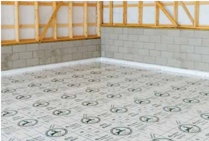
EPS in the foundation. PHOTO COURTESY OF HERSHEY'S METAL MEISTER
