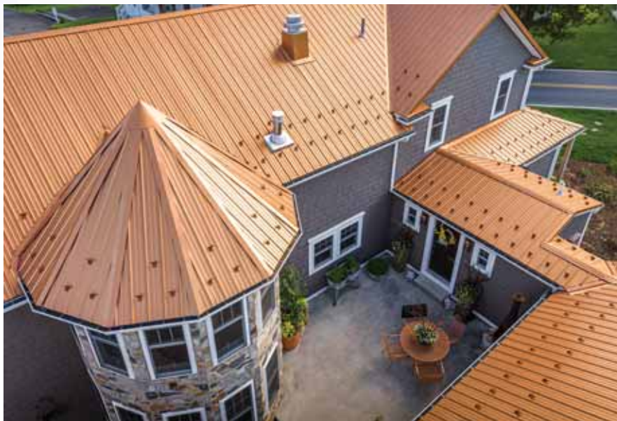
This beautiful copper roof shows the proper, staggered snow guard spacing. PHOTO COURTESY OF A.B. MARTIN
