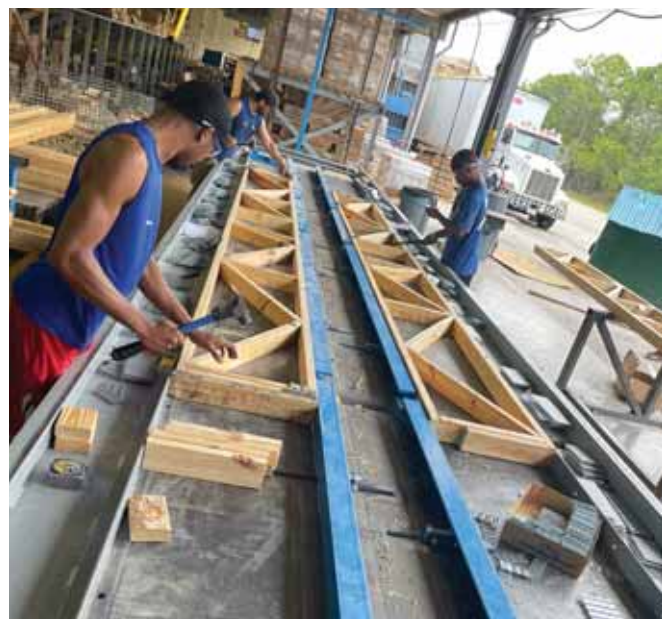
(BELOW) Pre-fabrication at the Plant. PHOTO COURTESY OF A-1 INDUSTRIES
