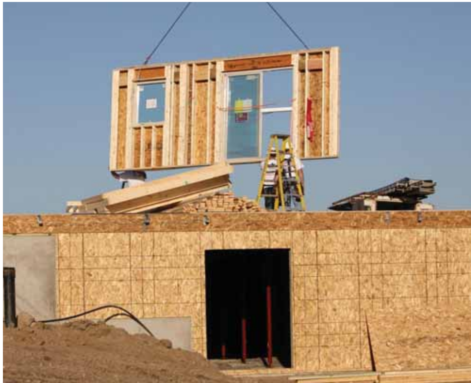
Wall Panel placement. PHOTO COURTESY OF DREXEL BUILDING SUPPLY
