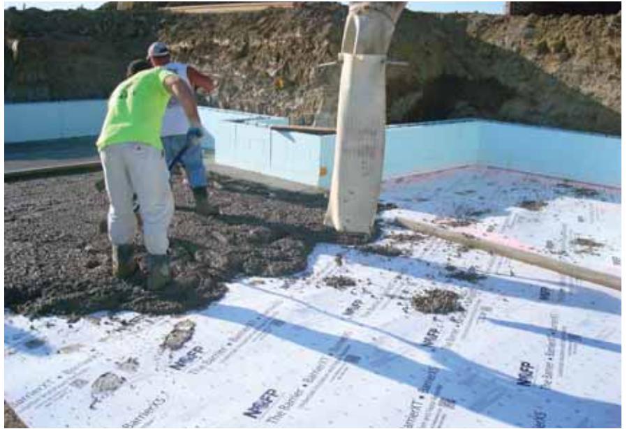
(RIGHT) EPS used beneath a concrete slab. PHOTO COURTESY OF NOFP
