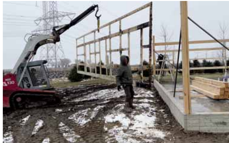
The Rapid Framing System can be placed with a telehandler or skid steer. PHOTO COURTESY OF H&D QUALITY BUILDERS
