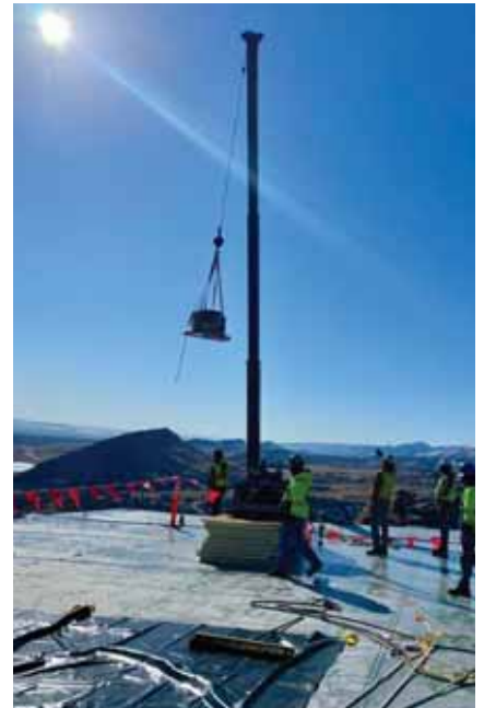
PHOTO COURTESY OF SUPERIOR ROOFING
