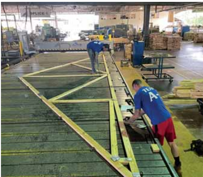
Pre-fabrication at the Plant. PHOTO COURTESY OF A-1 INDUSTRIES
