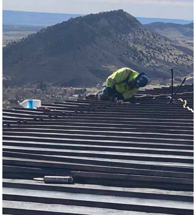
PHOTO COURTESY OF SUPERIOR ROOFING
