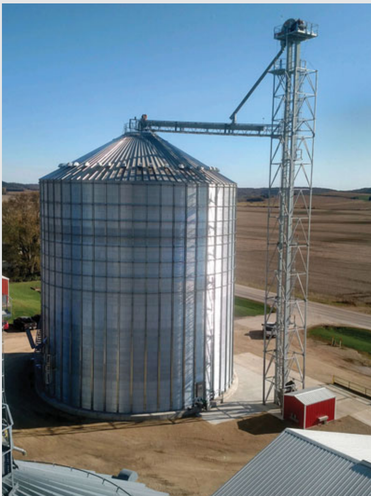
PHOTO COURTESY OF JAY CARPENTER
