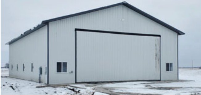
PHOTO COURTESY OF COVER'S CONSTRUCTION LLC.
