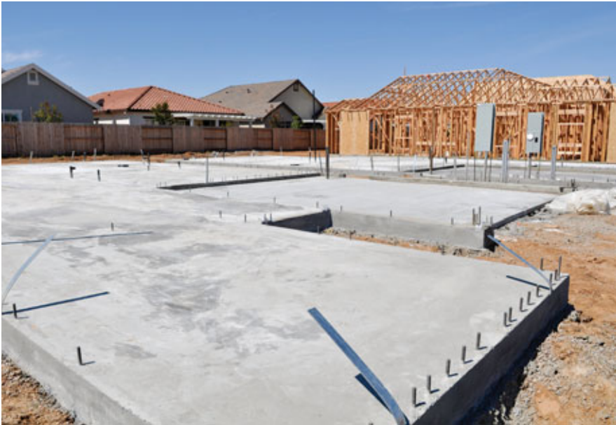
Concrete foundation for a house.
