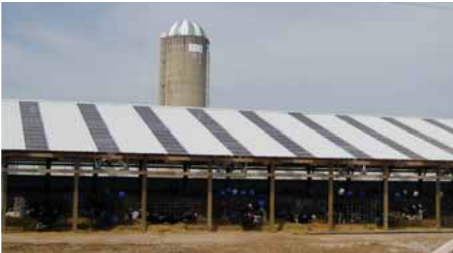
AmeriLux panels alternatively stripped into a metal roof.
