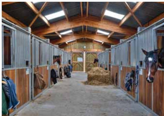
Barns, especially those for horses, are prime candidates for daylighting because of the benefits of natural light. PHOTO COURTESY OF AMERILUX.
