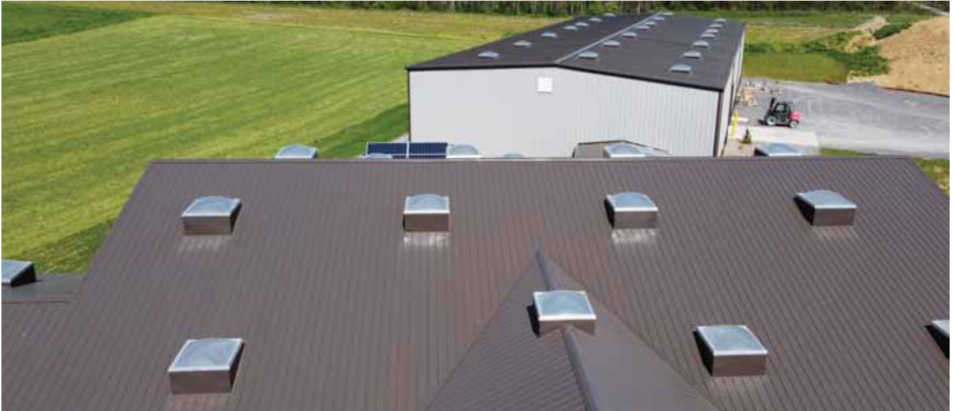
DayStar Natural Lighting Skylight Systems at work on a metal roof. Owner Kenneth Schlabach explained that these products have four parts: The dome at the top, roof curbs (the raised-metal frames that penetrate the roof), the light shaft, and the ceiling lens (on the ceiling, inside).
