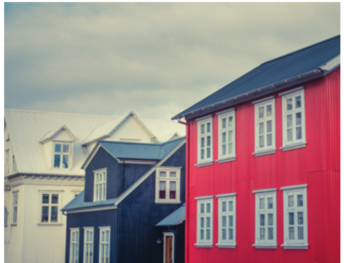
Traditional corrugated ironclad houses on a street in Reykjavik.
