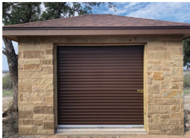
Shed with Sheet Door
