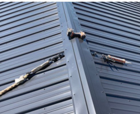
Ridgeline’s Safety Anchor has variations for all roof types and is virtually invisible while providing a tie-off point for life.
