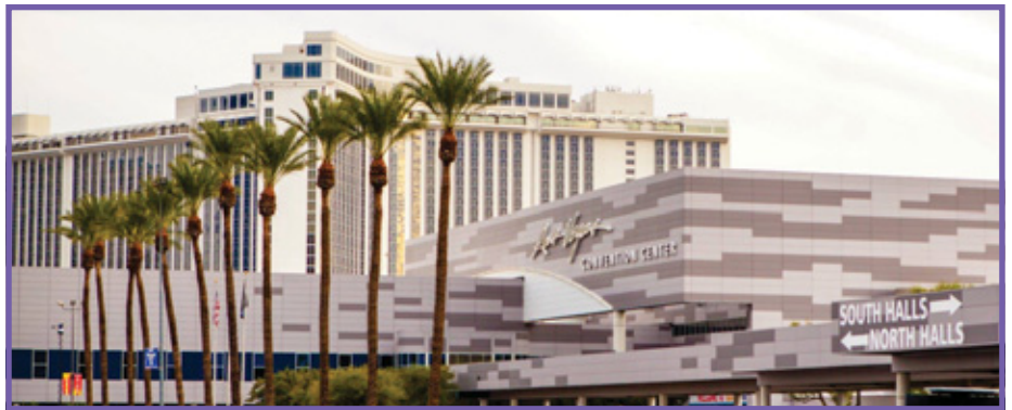
METALCON returns to the Las Vegas Convention Center in October. PHOTO BY MCOBAT PHOTOGRAPHY
