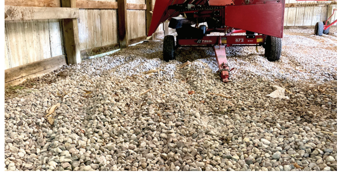
Using the same size of stone can result in rutting like this.
