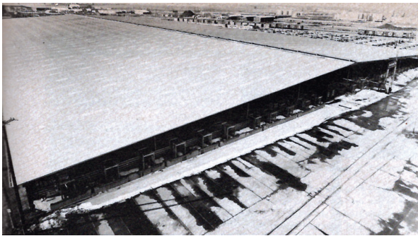
Largest and most modern facility of its kind, the Sioux City stockyards has this building covering 12.1 acres. Rainwater is collected from the roof and diverted to the river.
