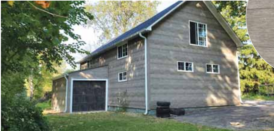
Western States Metal Roofing project.
