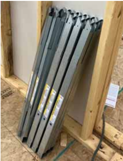
Top left: A truss being lifted onto the multi-family project in SE Wisconsin. This truss set took four hours, two hours less than typical. Above: For convenience and ease of shipping, handling and storage, the angled leg of a TrussBRACE can be folded flat. Top right and middle right: Workers setting trusses only from the bottom chord. Bottom right and below: Adding the TrussBRACE before the next truss is placed will save time and gives the framer something to do while they wait.
