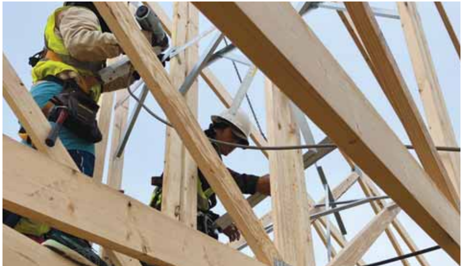
Top left: A truss being lifted onto the multi-family project in SE Wisconsin. This truss set took four hours, two hours less than typical. Above: For convenience and ease of shipping, handling and storage, the angled leg of a TrussBRACE can be folded flat. Top right and middle right: Workers setting trusses only from the bottom chord. Bottom right and below: Adding the TrussBRACE before the next truss is placed will save time and gives the framer something to do while they wait.
