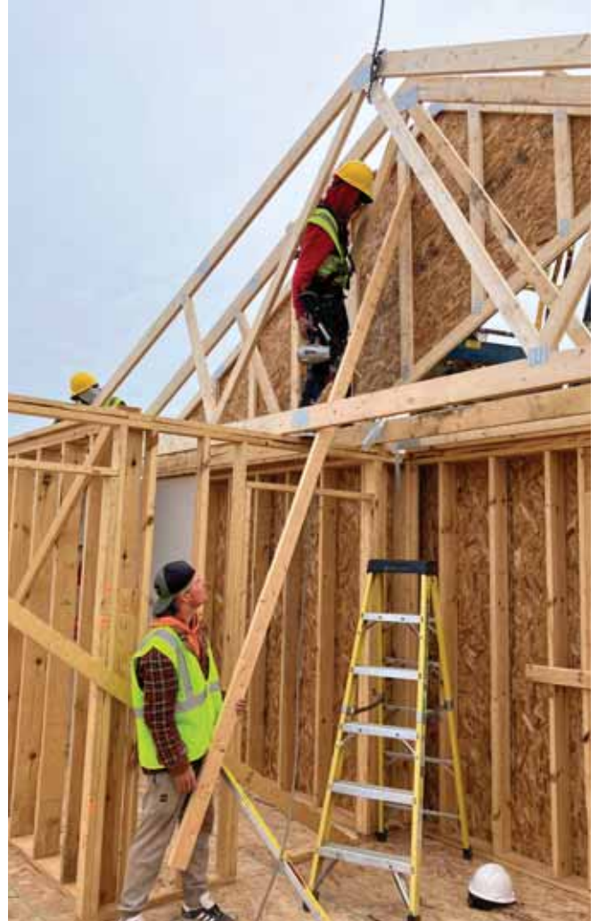
Nate Fischer (bottom) helps a framer get a truss in position.
