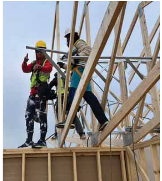
Top left: A truss being lifted onto the multi-family project in SE Wisconsin. This truss set took four hours, two hours less than typical. Above: For convenience and ease of shipping, handling and storage, the angled leg of a TrussBRACE can be folded flat. Top right and middle right: Workers setting trusses only from the bottom chord. Bottom right and below: Adding the TrussBRACE before the next truss is placed will save time and gives the framer something to do while they wait.
