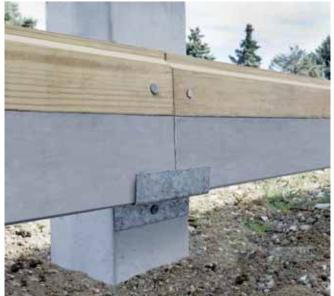
The industry's first patented precast concrete skirt board brought to you by Perma-Column. PHOTO COURTESY OF PERMA-COLUMN
