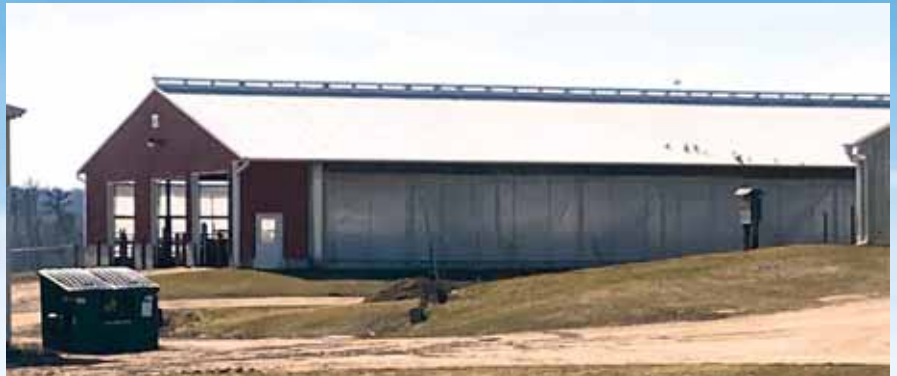
A high value or more sensitive operation on the farm (think babies) might dictate greater control and a more active system, while a less sensitive livestock population (adults or larger animals) or life stage might allow for a passive or natural ventilation system.
