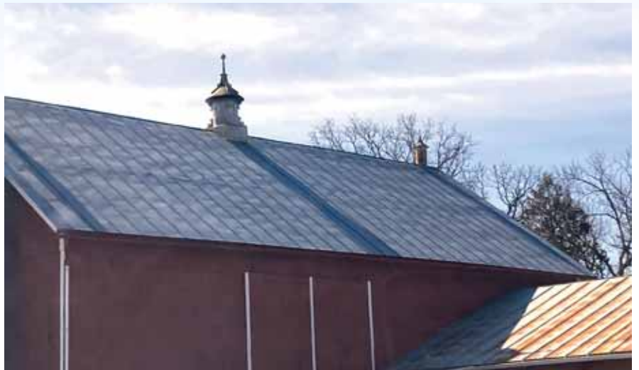
Old barns with cupolas show one of the ways that ventilation was used in multiuse (hay storage, animals, equipment) buildings in the past. These old barns usually had only a few animals in them and were mostly for storage of equipment and hay, so they had relatively low ventilation requirements. Today's livestock operations often need a bit more.
