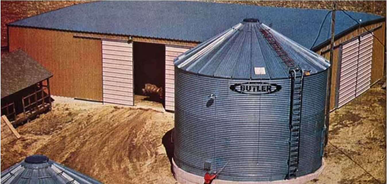
The Baumans needed a new machine shed and grain bin. Placing the bin adjacent to the machine shed, they could tap solar energy to dry grain.
