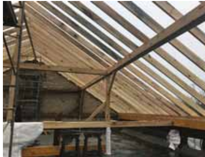
New timber framing just before sheathing is installed.
