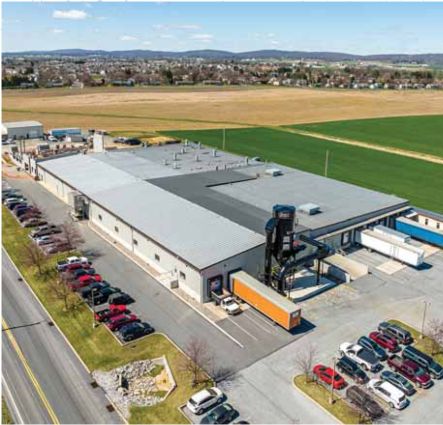
Lapp Millwright designed the dust collection system for Signature Custom Cabinetry's manufacturing facility.
