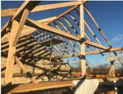
Timber framing progress on the north side.
