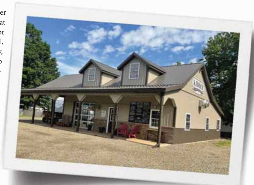
PHOTO COURTESY OF MITCHENER BUILDERS
