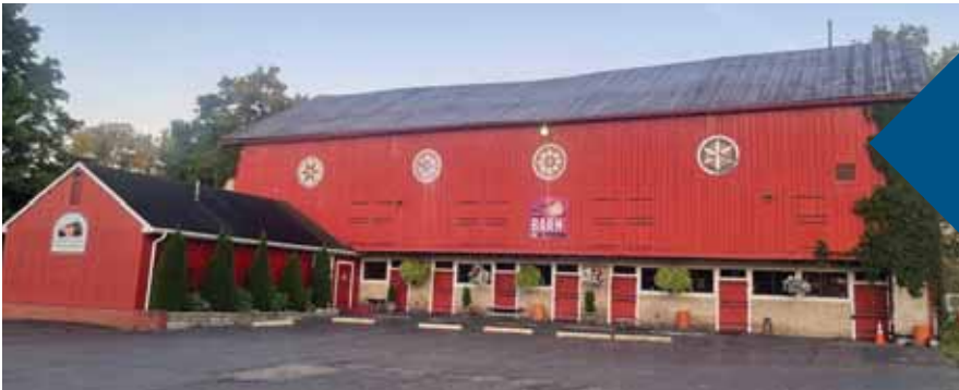
East elevation prior to Midstate beginning the roof restoration.
