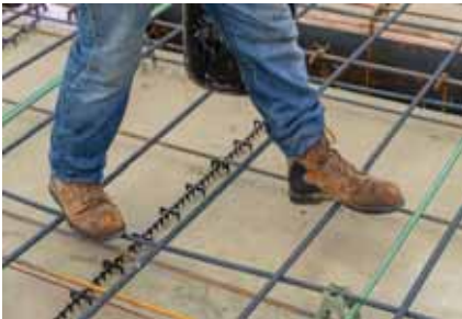
Sher-Bar TEC features enhanced bond strength with concrete compared to ECR, allowing grid congestion reductions and faster concrete pours compared to when using ECR.
