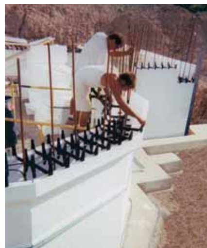
TechBLOC forms for the Buffalo house came in 16-in. x 48-in. panels, which are stacked and then spreaders and rebar are installed.
