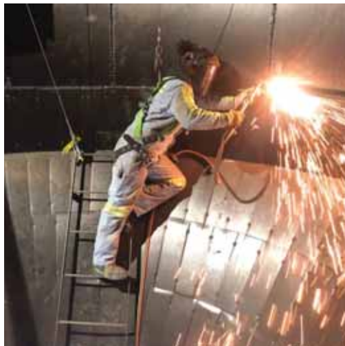
Sarah Jones cutting down the angle iron in an asphalt silo.
