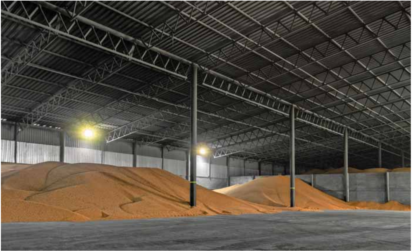
One option is to store grain on a concrete slab in a covered building. An advantage is that it can be a multipurpose structure for equipment storage as well.
