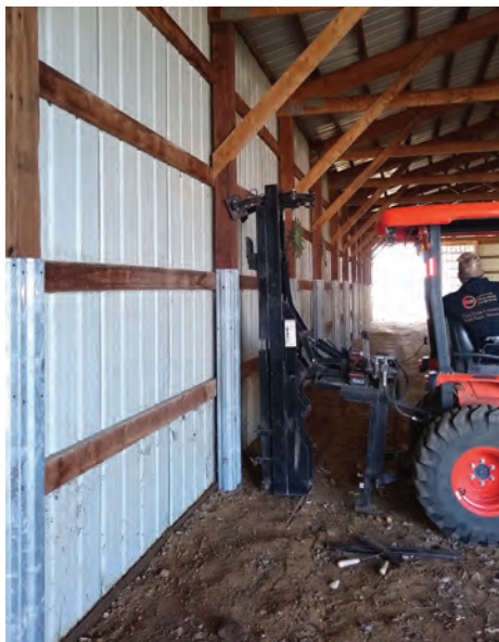
Repair Sleeves being installed.
