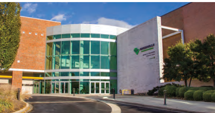
The Greenville Convention Center is the home to the 2025 Garage, Shed & Carport Builder Show.
