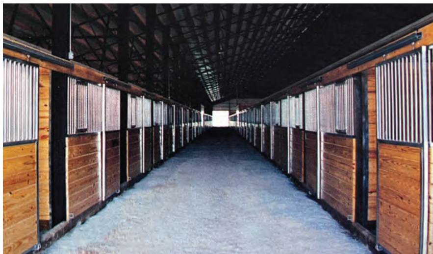
A fine, white stone provides the finished surface of the aisles, which separate back-to-back stalls in the center and larger foaling stalls along each perimeter of the building.
