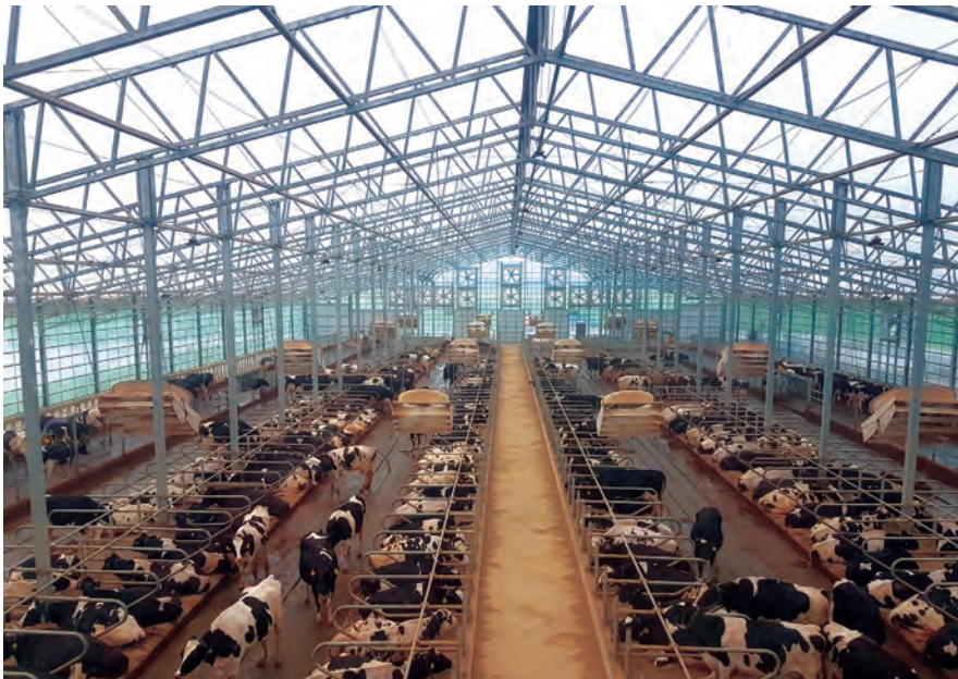
A major advantage of a tension fabric structure, like this one by WeCover, is that it allows natural light, which not only saves on lighting costs, but is good for livestock health.
