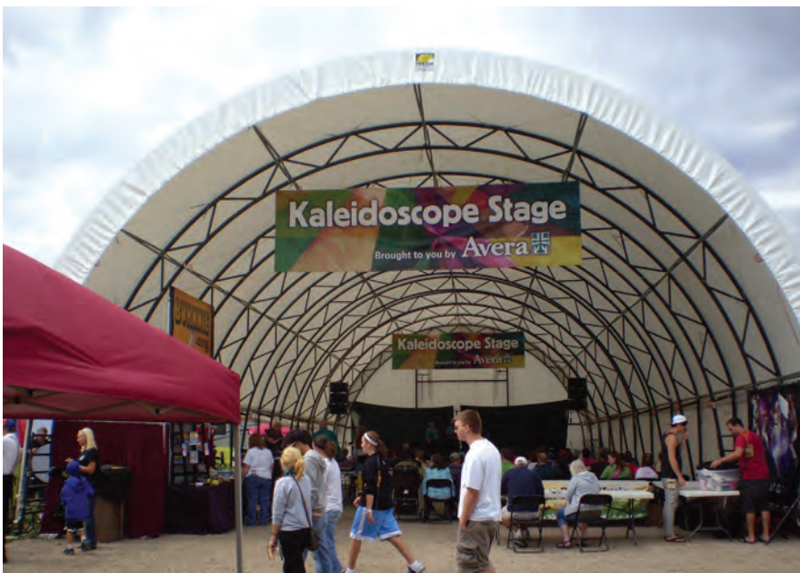
Tension fabric structures, like this Sioux Steel Pro-Tec Building, are ideal for temporary event and entertainment shelters, as they're sturdy and can be quite large, yet they can be erected and taken down relatively quickly. PHOTO COURTESY OF SIOUX STEEL.
