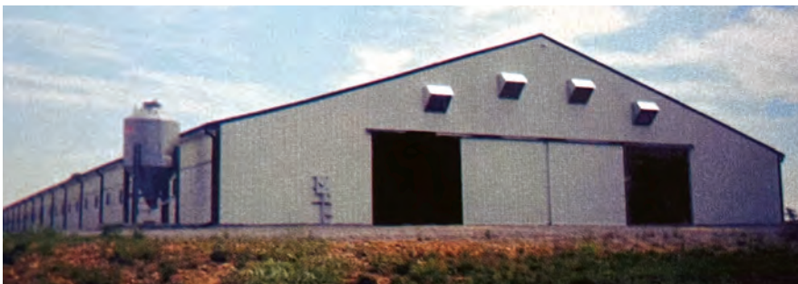
The finished mare breeding barn measures 96 ft. wide and 378 ft. long, housing 93 stalls; examining, surgical, and washing space for a veterinarian; and storage space for feed and hay.
