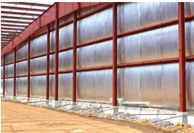
Thermal insulation, such as fiberglass batting, reduces heat transfer primarily through conduction and convection, whereas reflective insulation (like that insulation seen above), reduces heat transfer by reflecting radiant heat.
