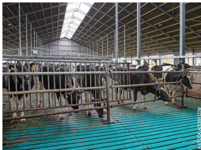
This livestock building has excellent natural lighting, adequate space for the cows to move freely, and slatted floors that are easier to keep clean than solid concrete floors.
