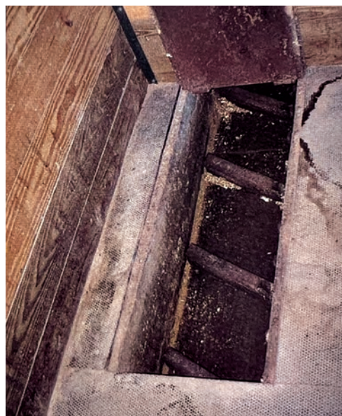
The manure conveyor system at Carriage Ridge allows stalls to be cleaned quickly, and the manure plowed in to the soil.
