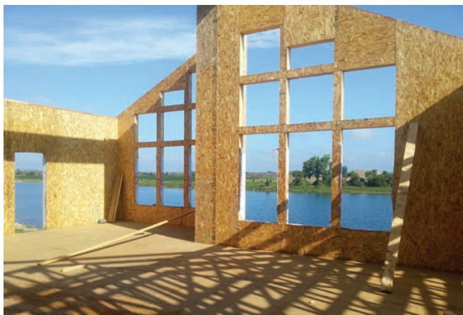
A SIP building's self-contained panels make building much faster than conventional stick-built construction, as fewer pieces and steps are needed. PHOTO COURTESY OF SIPA.
