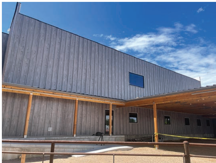
(Left) Lee Smith used a New Tech Machinery portable roll former to form the printed steel board and batten panels on this building called The Legacy Project. PHOTO COURTESY OF NEW TECH MACHINERY.
