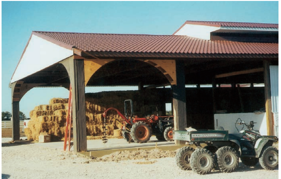
Tile on a pole barn? Post-frame structures nearly always feature metal roofs, but they don't have to be ribbed panels. This 18,000-sq. ft. horse barn in Weimar, Tex., shown here under construction, ended up with half-stucco walls and a tile roof — metal tile, that is. "It cost us more than a regular panel, but this is our office, and we wanted something unusual," says Sharon Duperier of Legacy Building Systems. "It's a real show-stopper." The long panels from Met-Tile weigh only 125 lbs. per square and easily meet the structure's wind loading requirements. MET-TILE PHOTO
