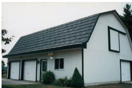
Wood-grained and granular-coated Woodland metal shingles from Dura-Loc spruce up this plain utility building without sacrificing the low maintenance and durability expected for such roofs. DURA-LOC PHOTO
