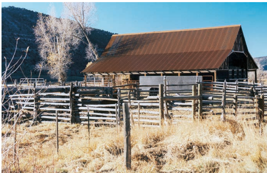
In arid climates, the beauty and surprising longevity of rusted metal has led some to use unpainted and uncoated steel on roofs and sidewalls. This barn in southern Colorado sports rusting, cold-rolled carbon steel panels from Recla Metals in Montrose, Colo. "Weathering steel," known by its US Steel trade name CorTen, can give a similar rusted look with greater longevity, but at a steeper price. RECLA METALS PHOTO
