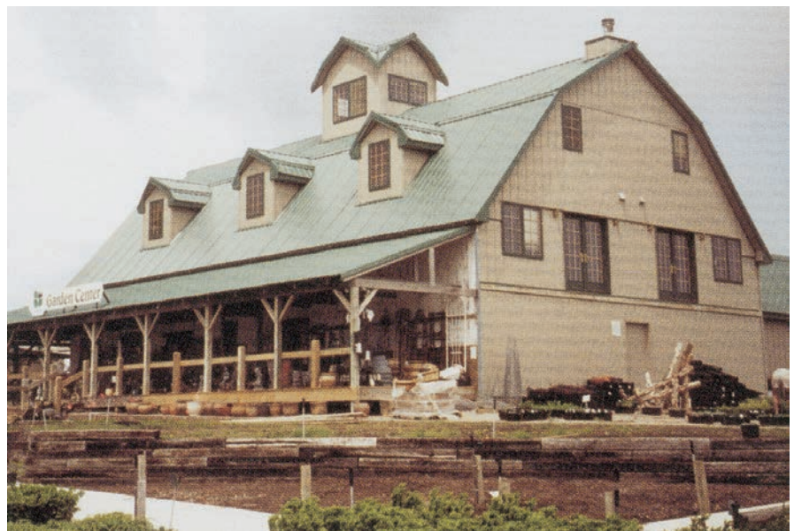
"Ag panel," the standard 36-in., 29-ga. painted G90 ribbed panel, and other screw-down profiles have a reputation as inexpensive but drab and industrial. But that's largely a matter of where it ends up. It may look homely on the side of a windowless machine shed, but the same material nicely spruces up this gambrel-roofed barn with dormers. The right color and an interesting roofline make the difference. DURA-LOC PHOTO
