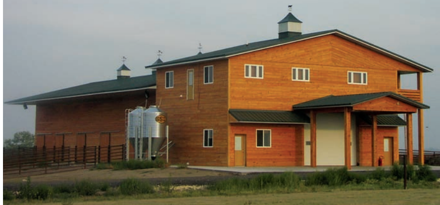
Kansas builder Wes DeBey built this 5,300-square-foot combination bull barn/living quarters using ICFs, chosen for their sound proofing ability. REWARD WALL SYSTEMS PHOTOS
