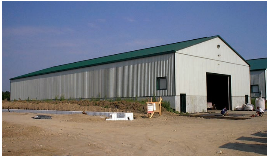
With added rebar, the ICF walls of Bert Tupling's potato barns withstand the weight of the 5.5 million pounds of potatoes he piles 19 feet high in each building. ARXX BUILDING PRODUCTS PHOTO
