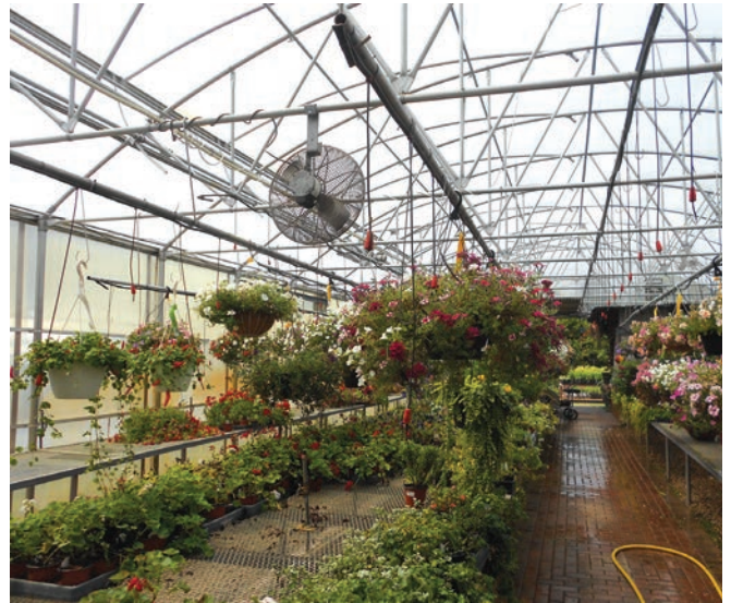
Strategically positioned fans circulate air to help regulate ventilation in this greenhouse operated by Chain O Lakes Home and Garden in Waupaca, Wisconsin. SHIELD WALL MEDIA PHOTO.
