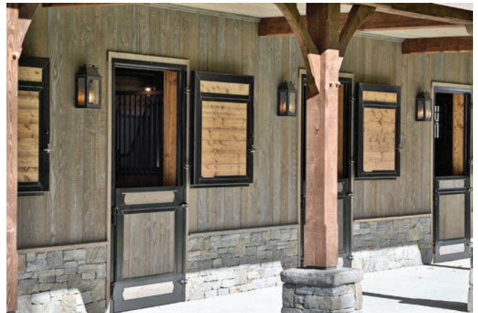
Exterior Dutch doors not only provide horses fresh air but also both horses and their human caretakers an alternate way to escape in case of a barn fire. Given a barn’s wood construction and the hay and other flammable materials they contain, the risk of a rapidly spreading fire is a real concern. PHOTO COURTESY OF WINTERFELL FARMS AND CLASSIC EQUINE EQUIPMENT
