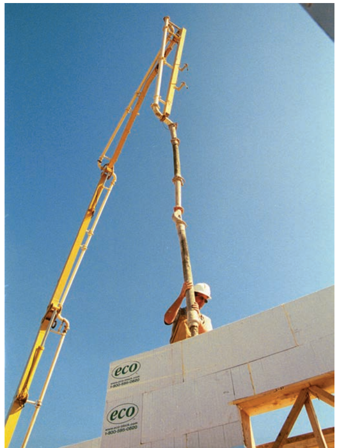
Insulating concrete forms, long used in residential projects, have been gaining popularity for use with agricultural buildings.
