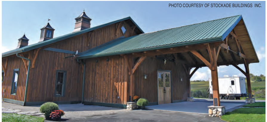
PHOTO COURTESY OF STOCKADE BUILDINGS INC.
