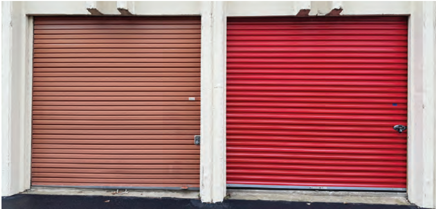
Worn storage facility unit on left. Renew-Rite refreshed unit on right.
