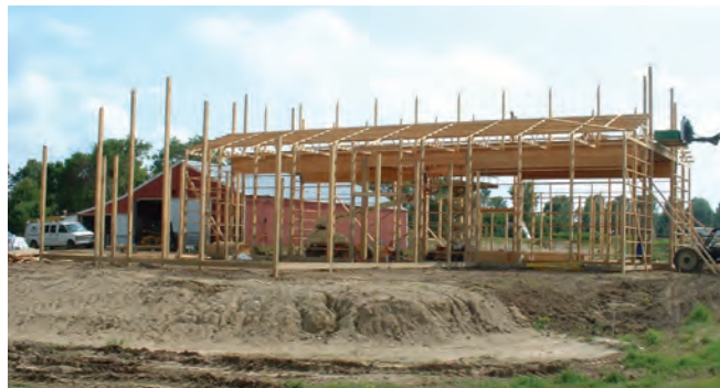
D&W Construction designed a second floor for hay storage, as well as an opening for future installation of a lift.
