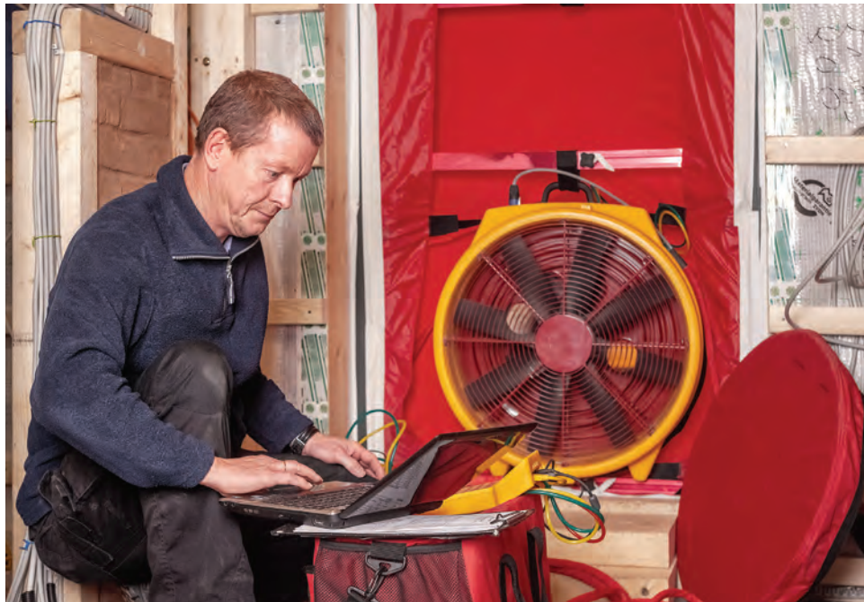
A blower door test works by mounting a special fan in an exterior doorway to check how airtight a building is. All exterior doors and windows are closed, and interior doors are left open so air can move freely. The fan either pulls air out or pushes it in to create pressure, which helps pinpoint where air is leaking through cracks or gaps in the structure. INGO BARTUSSEK-STOCK. ADOBE.COM
