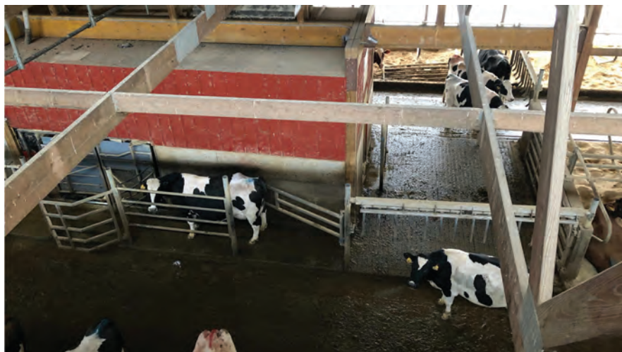
It is essential that AMS facilities be designed for one person to move cattle easily and efficiently around the robot with the least amount of stress. COURTESY OF THE DAIRYLAND INITIATIVE.
