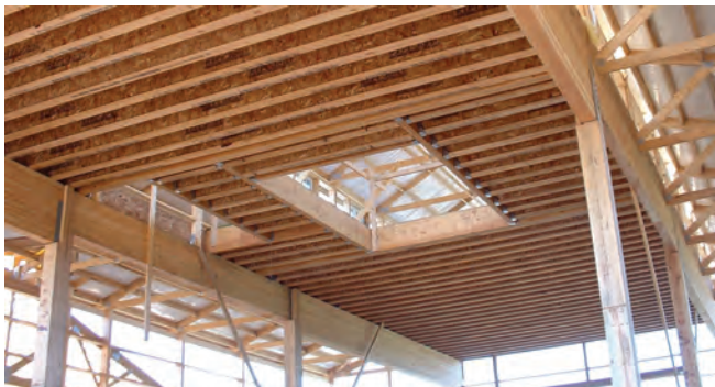
D&W Construction designed a second floor for hay storage, as well as an opening for future installation of a lift.
