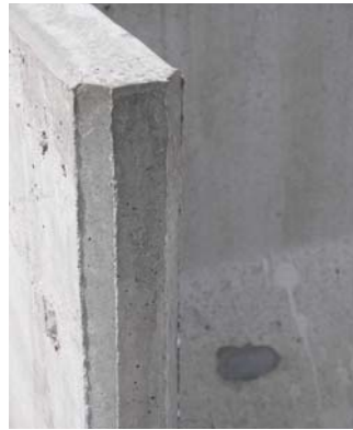
▲ Corners at walk-throughs were rounded at Eron's request for cattle safety so cattle could be moved in and out of pens without injury or bruising.
