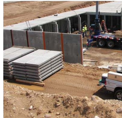
▲ Corners at walk-throughs were rounded at Eron's request for cattle safety so cattle could be moved in and out of pens without injury or bruising.
