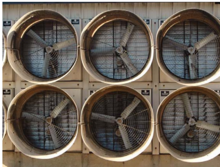
ABOVE Tunnel ventilation systems are popular for poultry, swine and dairy barns. The fan banks shown above help to ventilate a large dairy operation located in eastern Wisconsin.
