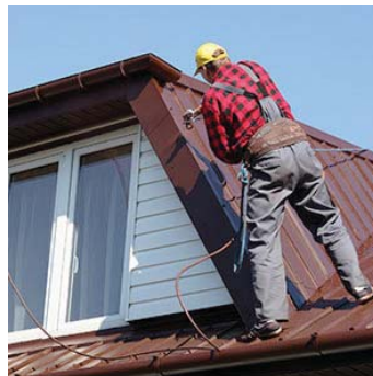
Installation of WeatherXL Crinkle Finish. Photo courtesy of Valspar
