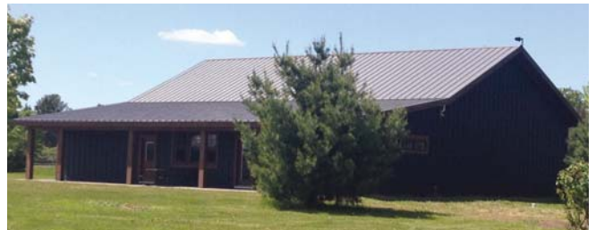
Metal was used on this New Auburn, Wisconsin, building to save on the maintenance typically needed for wood-frame structures.
