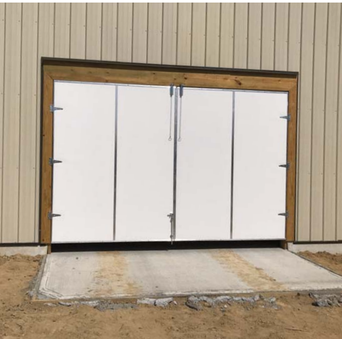
5. These broiler houses on the Delmarva Peninsula, Delaware, feature large poultry end doors from Plyco. For ease of maneuverability, they are made of aluminum. The smaller walk doors are steel and are also made specifically for the ag industry. All doors have steel hardware. Photo courtesy of Northeast Agri Systems.
