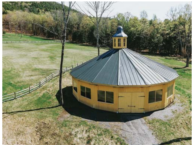
Rofer John Kinnarney of Iron Horse Roofing used patience and Englert S2500 steel panels for the roofing.
