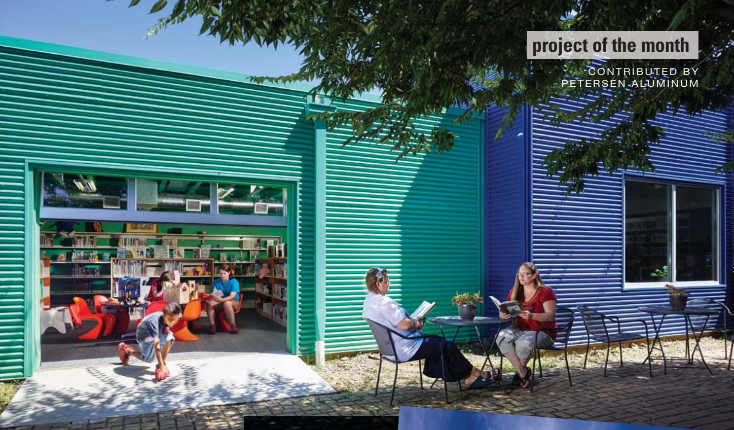
The low-maintenance of metal was a major selling point for this project. Photo credit: Petersen Aluminum
