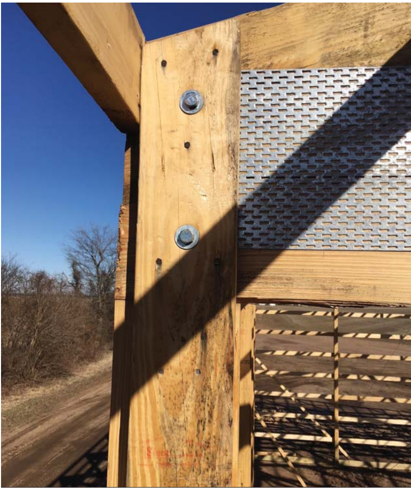
PICTURE 2. Bolted connection of truss to a 3-ply laminated column resists rollover of the heel during construction. Photo courtesy of Stockade Buildings Inc.
