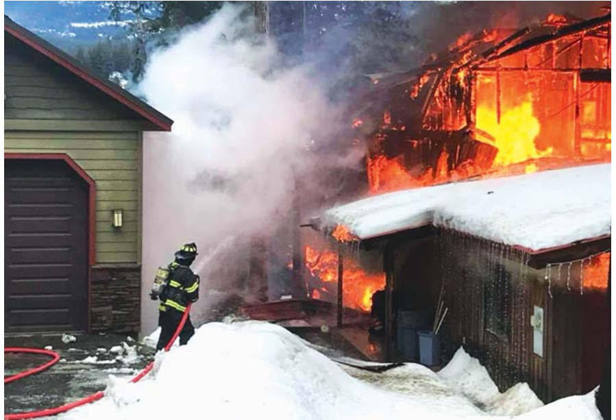
The home on the left withstood extreme heat from a neighboring fire. Its HardiePlank fiber cement siding was credited with saving it. Photo courtesy of James Hardie Industries
