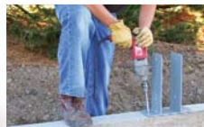
Sturdi-Wall™ Brackets Drill set for cured foundations
