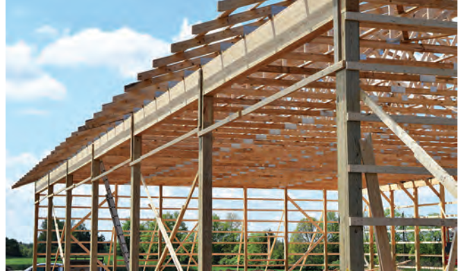
Booth 536: Rigidply Rafters Glulam Posts.
