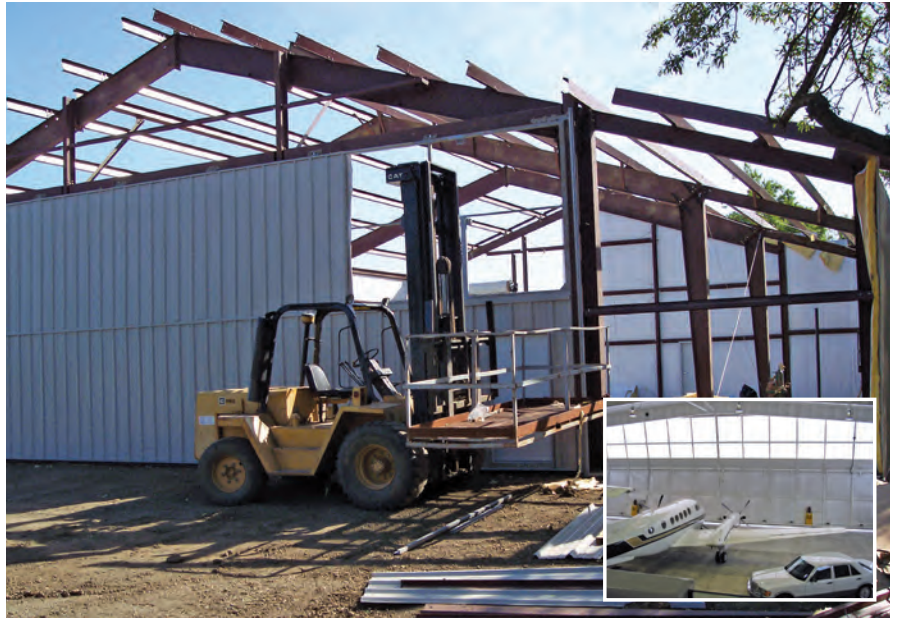
BC Schmidt Construction of Williams, Calif., specializes in building airplane hangars, a fast-growing market. “There are so many fun things, so many exciting things you can do with a hangar,” says Carrie Schmidt. BC SCHMIDT CONSTRUCTION PHOTOS
