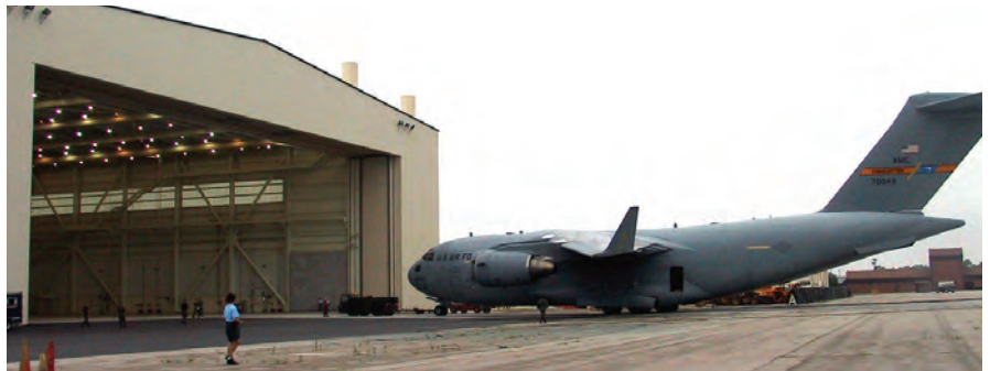
There’s always room for mega-hangar jobs: South Carolina builders Hightower Construction presided over this C17 hangar at Charleston Air Force Base. BUTLER HEAVY STRUCTURES PHOTO
