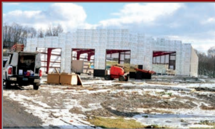
Thermal 3Ht WRE 1 inch only on walls & roof directly on frame and RRE 1/2 inch only under radiant heat floor!
