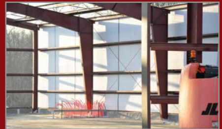
Thermal 3Ht WRE 1 inch only on walls & roof directly on frame and RRE 1/2 inch only under radiant heat floor!
