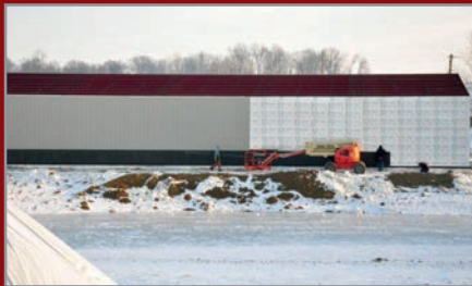
Thermal 3Ht WRE 1 inch only on walls & roof directly on frame and RRE 1/2 inch only under radiant heat floor!
