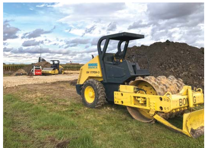
Site prep and foundation work for a two-building, 20,000 sq. ft. climate-controlled storage building expansion. Planning for stormwater handling and underground utilities for current and future phases is an important part of self-storage development.
