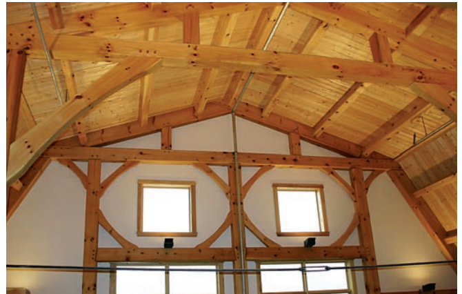
A spectacular gambrel entryway is sheathed with structural insulated panels. SCOTT TAPPA PHOTOS
