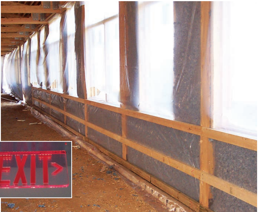
LED exit signs from Cooper Lighting are energy efficient, operating on 1.5 watts each. Ultra-Touch insulation from Bonded Logic is made from recycled materials with no harmful chemicals, and has an impressive R-value.
