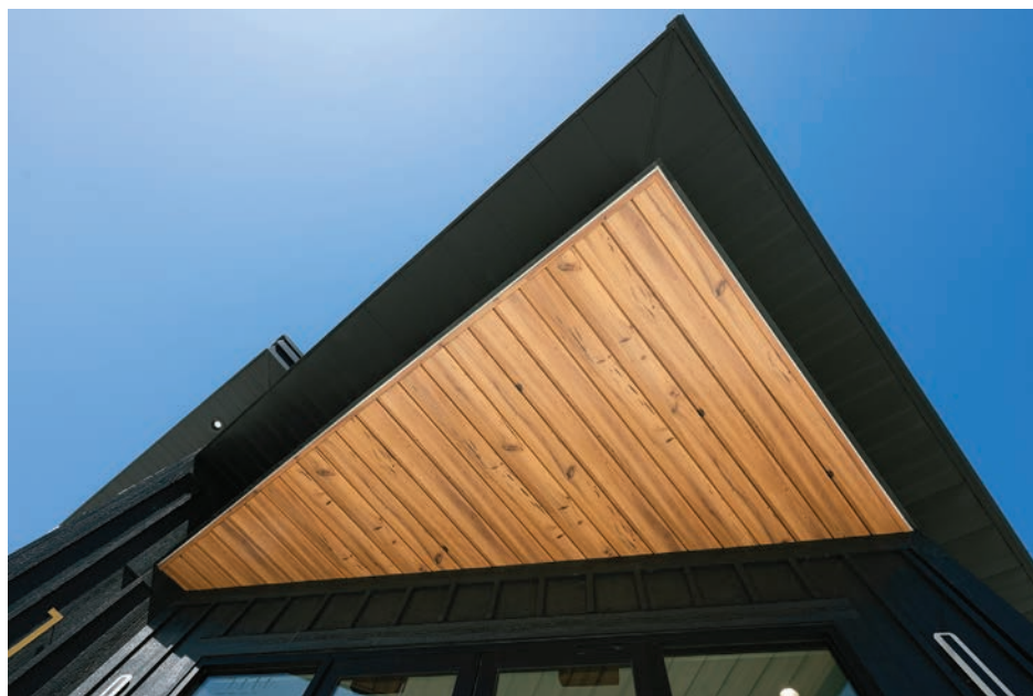
Tru-Steel HD® digitally printed steel, in a woodgrain pattern.
