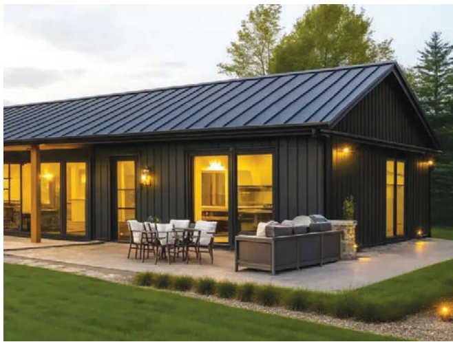
IMAGE COURTESY OF ELITE BUILD COMPANY
