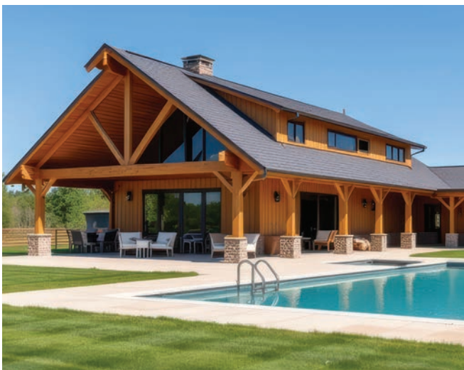
IMAGE COURTESY OF ELITE BUILD COMPANY
