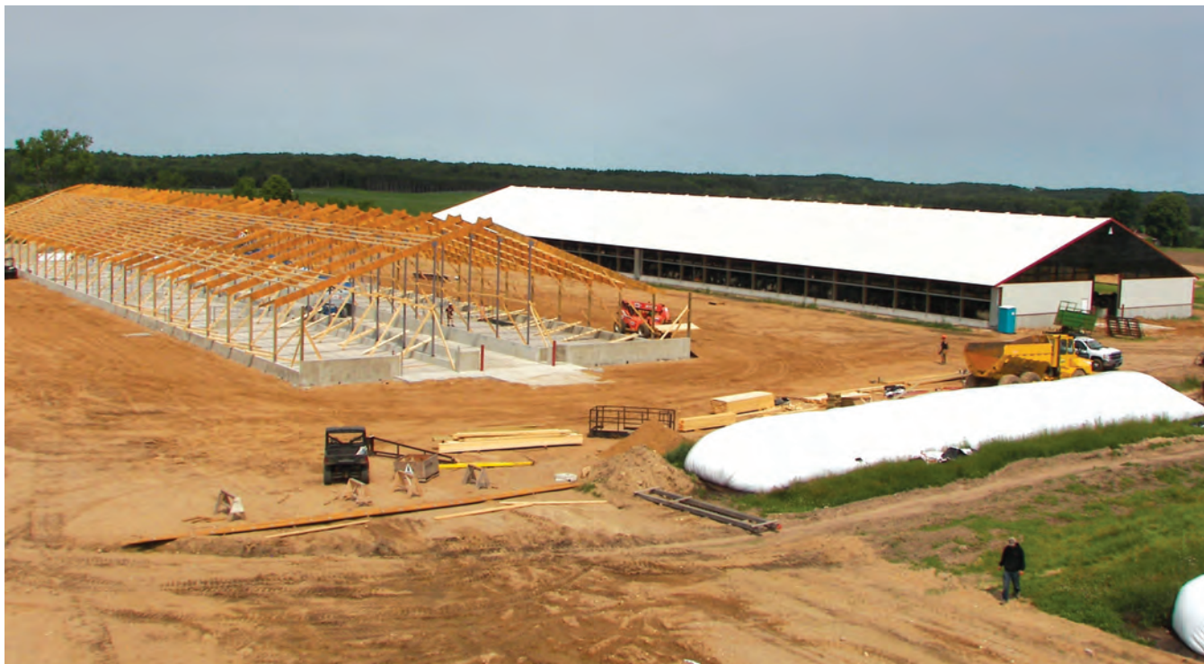
Owner Dave Eron now operates Eron Beef LLC out of two new post-frame barns, both completed in 2015, near Stevens Point, Wisconsin. The calf barn is under construction in this photo. The finishing barn is to the right.
