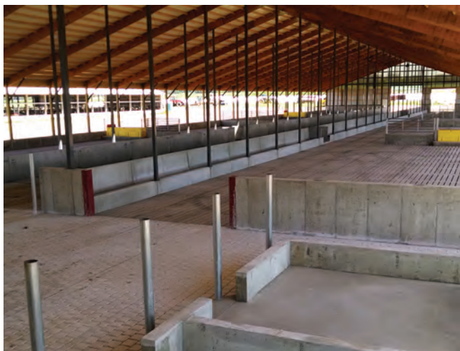
The last three bays of calf barn (36' X 90') are reserved for working facilities and an office and utility room.
