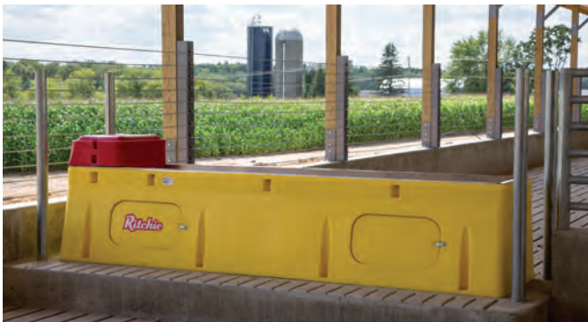
Cattle drinker pads and plumbing were constructed so as not to interfere with the pit below.
