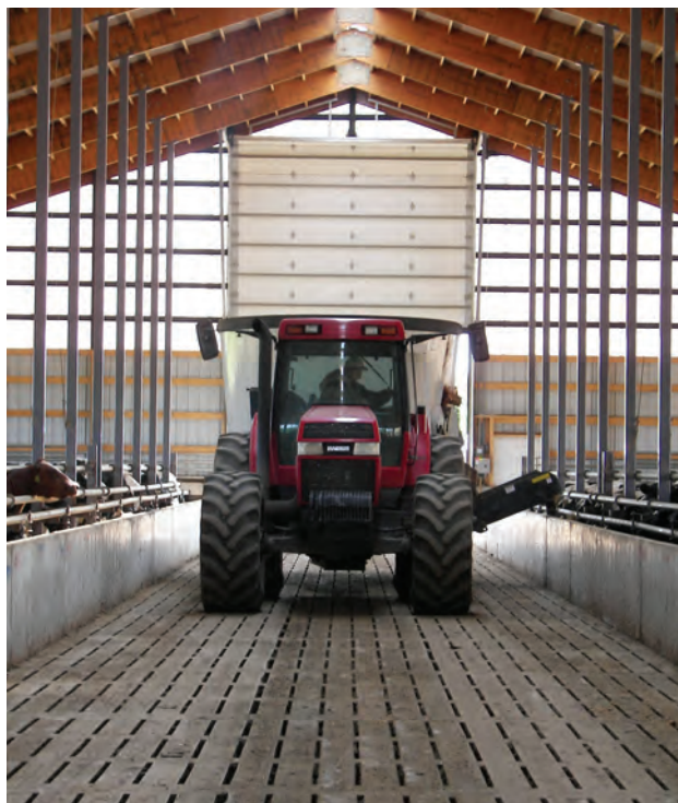
T Feeding is done inside the barn thanks to extra pillars built in the manure pit to allow for heavy traffic above.
