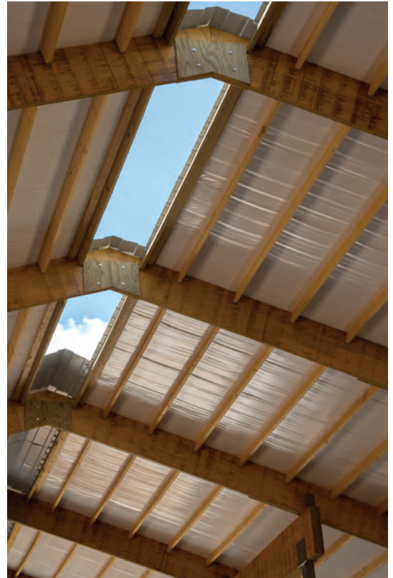
(Eron discovered that an open-ridge roof is an economical option for naturally vented, slatted floor livestock barns like his.
