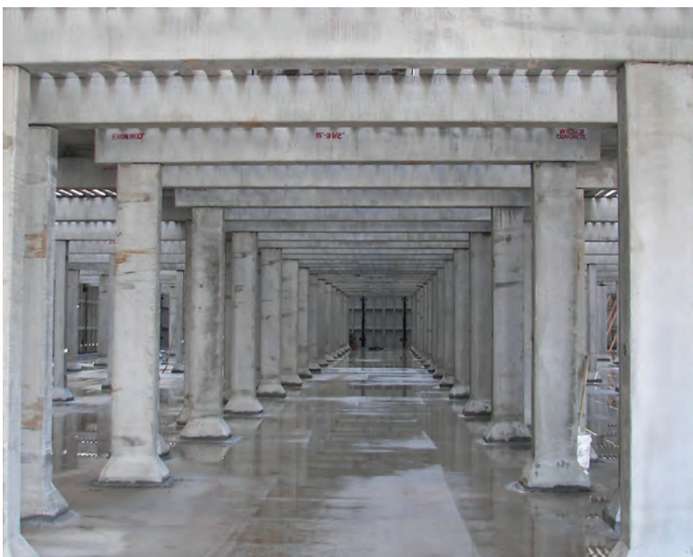
Wieser Bros. Concrete erected the pre-cast, 12-foot deep pit over a 6-inch poured Ready-Mix floor. Eron wanted drive-through feeding inside the barn, so extra posts and support beams in the pit allow for more strength above for heavy equipment.
